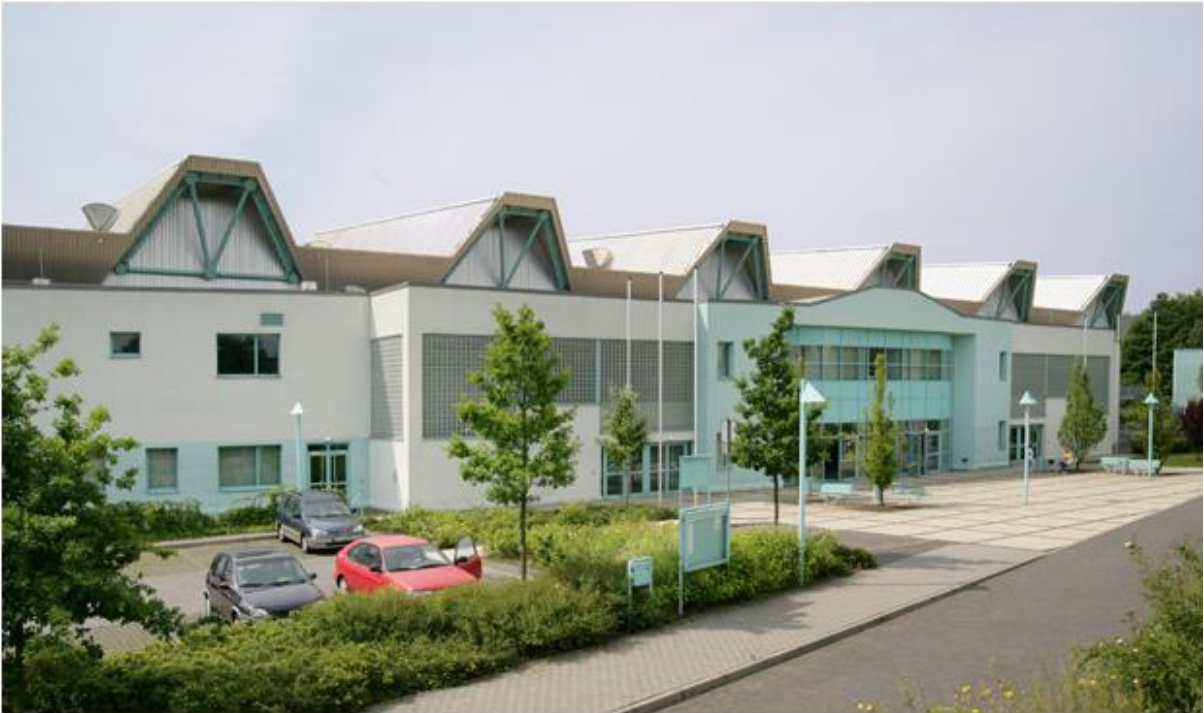
Picture 1: View of the Gymnasium Brandberge Halle (Saale).
